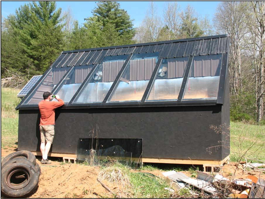
Figure 7. Solar kiln and solar-photovoltaic-driven fans.
