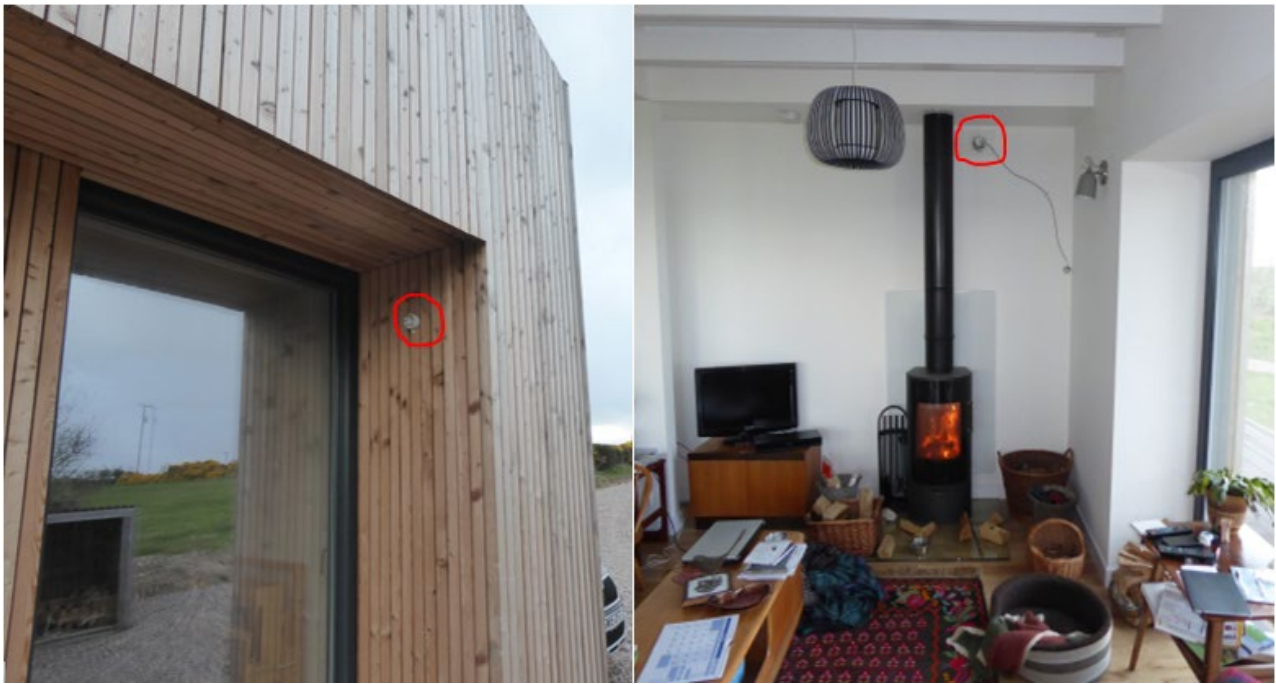
Fig. 10. Sample of performance monitoring sensor positions
