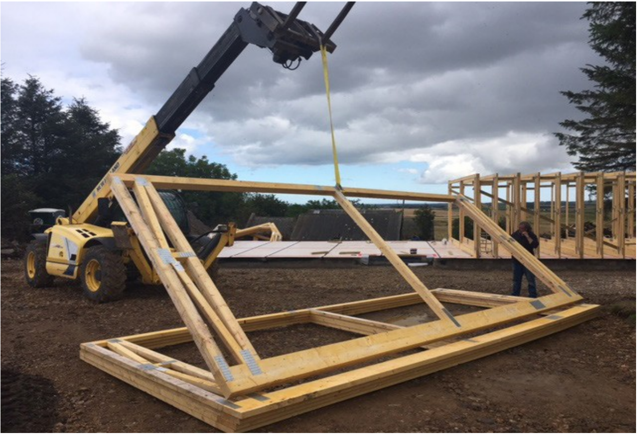
Fig. 4. Individual truss frames being put in place with light-weight machinery
