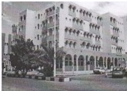
Figure 1 : An exterior view of the CNAS building showing its various openings.
