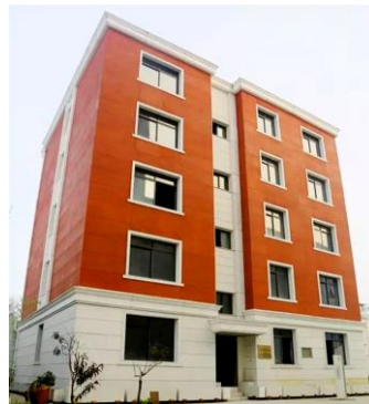
Figure 3. Winsun 6-Story tall 3D printed building
