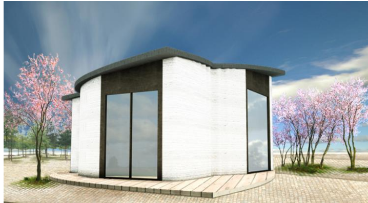
Figure 4. First 3D concrete printed building in Europe by COBOD
