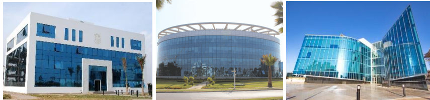
Figure 3. Office buildings in Cairo, Egypt with curtain wall façades facing west and south.
