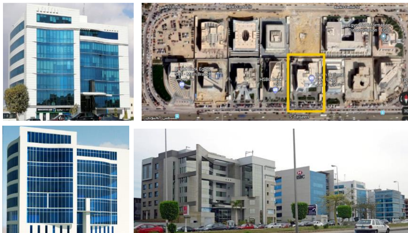
Figure 1. The site layout of the case study building, actual building shot and 3D model
