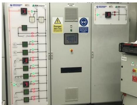
Figure 3: MaREI microgrid distribution panel
