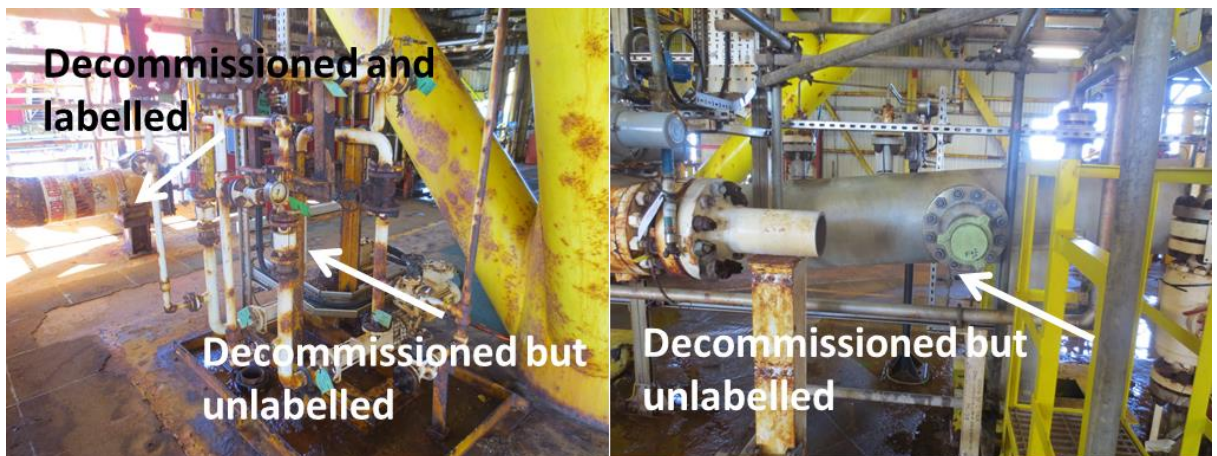
Figure 7-11: Poor identification of decommissioned equipment. Source: Author
