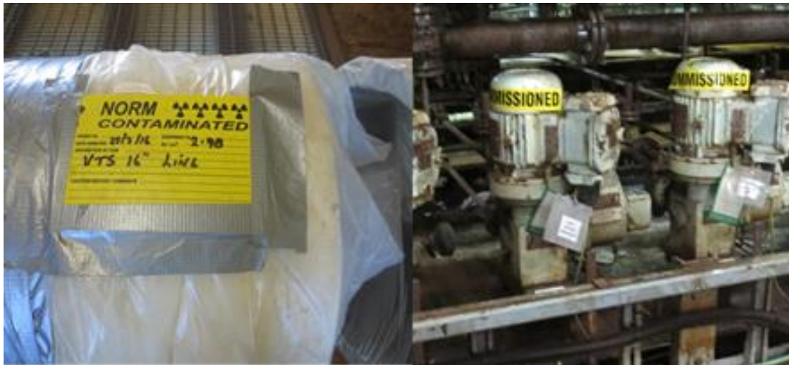
Figure 7-14: Improved marking of decommissioned equipment. Source: Author
