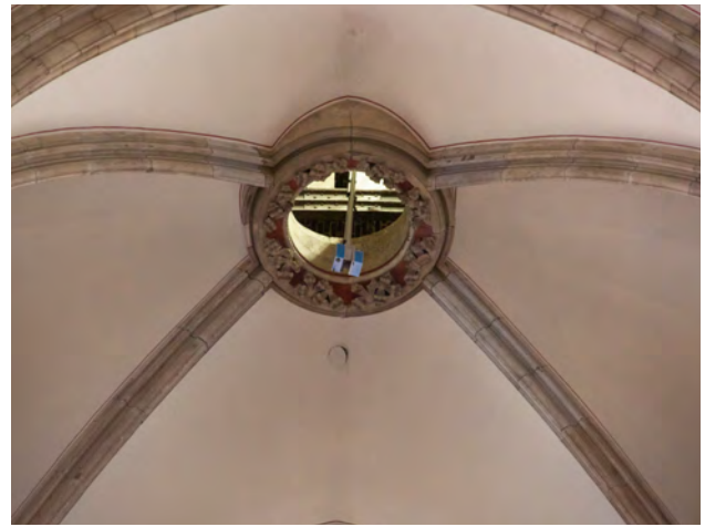
Image 5: The remotely operated, inverted 5010C TLS at the Cologne Cathedral.
