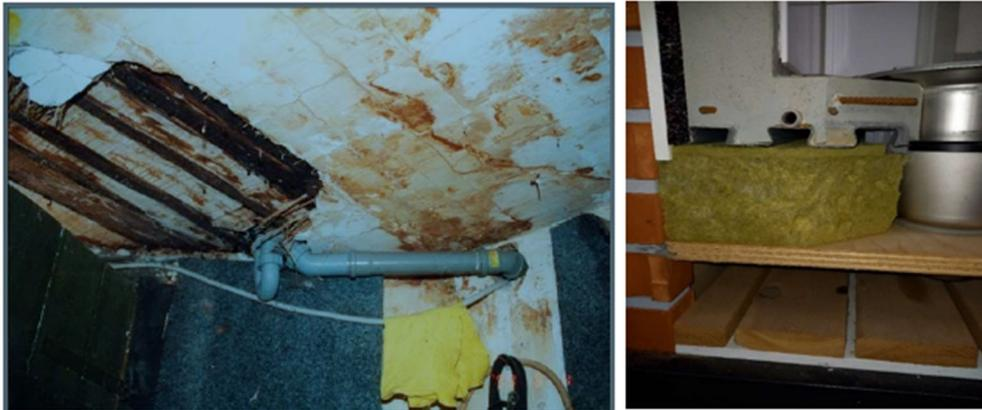
Figure 8. Wet room disaster, water penetrating from a bathroom above, where the membrane was omitted. Photo by the Author
