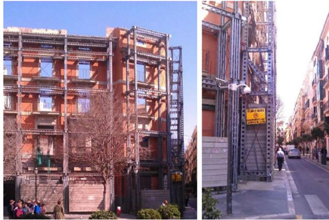
*Figure 10. Street façade in Palma de Mallorca, the brick façade has been kept to ensure the street environment, behind the façade, a new building will be fitted. Photo by PJA*
