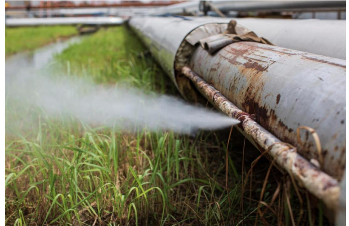
[1] – figure 1 – Corrosion Under Insulation Pipe Leak
