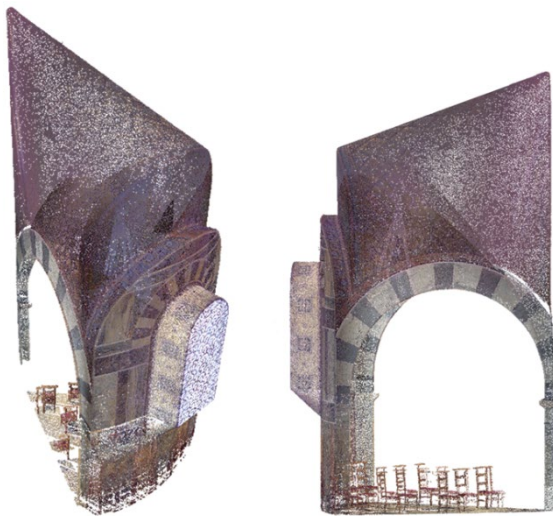
Figure 6. First-floor conic vault.
