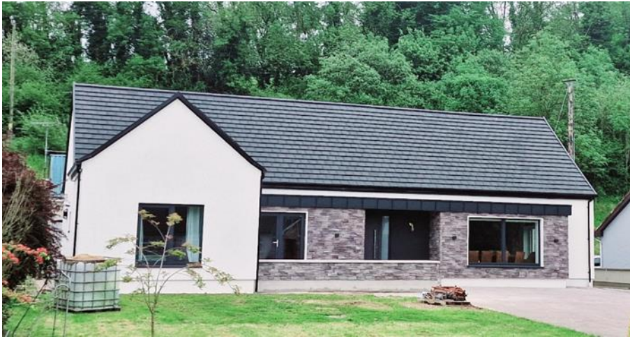
Figure 2. Bungalow after Retrofit.
