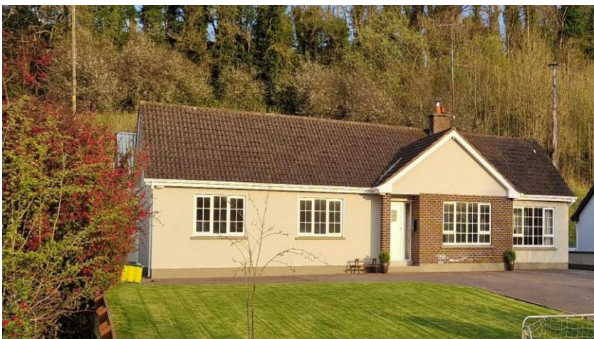
Figure 1. Existing Bungalow Before Retrofit.
