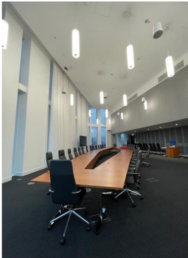
Figure 2. Meeting room and existing fire safety devices.
