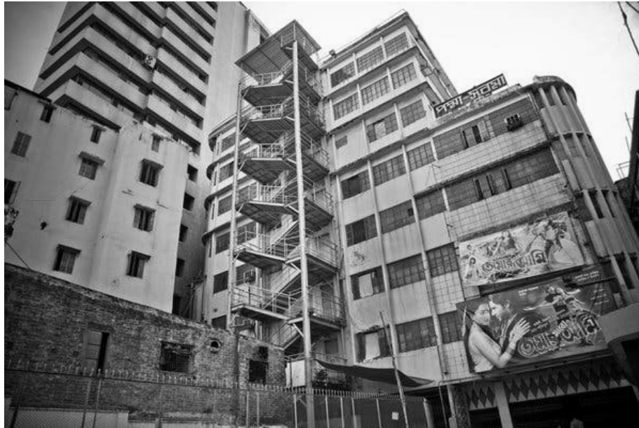
Figure 2: Complex juxtaposition of industry and residential building (source: Khaled Hasan for The New York Times, 2013 (accessed: After Disaster, Bangladesh Lags in Policing Its Maze of Factories - The New York Times (nytimes.com) on 14 January 2024)
