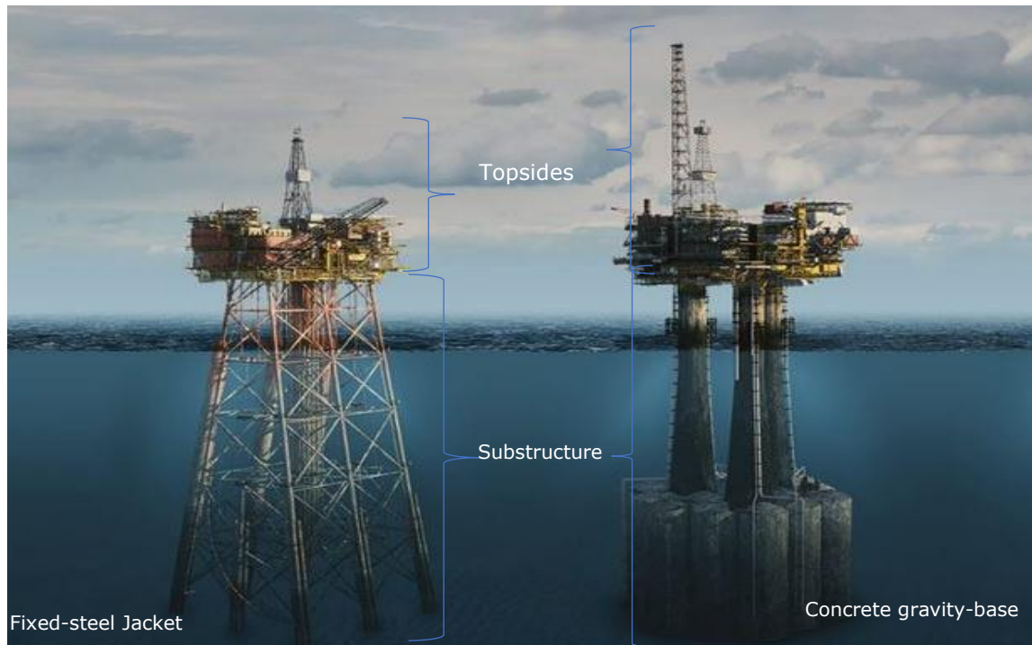
Figure 2.2: Components of an offshore platform (Adapted from Rachain 2017)
