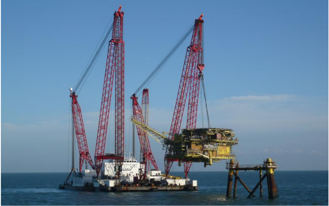
Figure 2.3: Removal of the Welland platform topsides (Nixon 2019)
