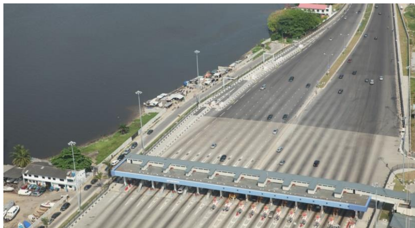
Aerial view of one of the completed Toll Plaza. Source: RCC (2022)
