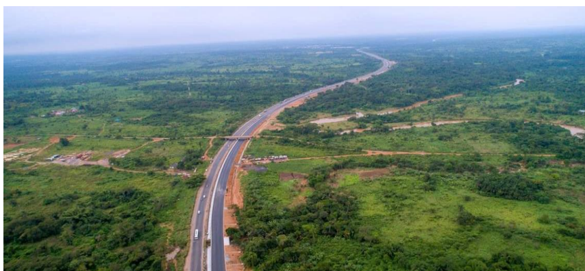
Drone aerial view of Lagos-Ibadan Section II highway project Source: RCC (2022)
