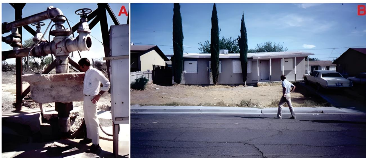
Figure 5. (A) the elevation of drill pipes and (B) the destruction of a house in the Windsor Park District caused by land subsidence [137].
