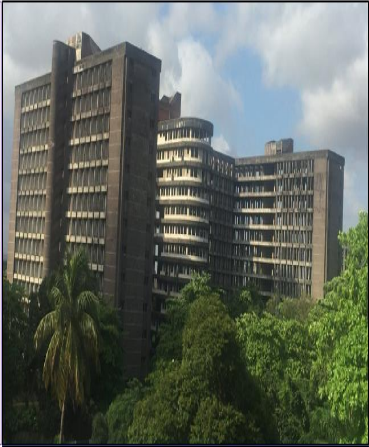
Case Study - Federal Secretariat - Alausa, Lagos, Nigeria (Source: Ayeyemi 2022)
