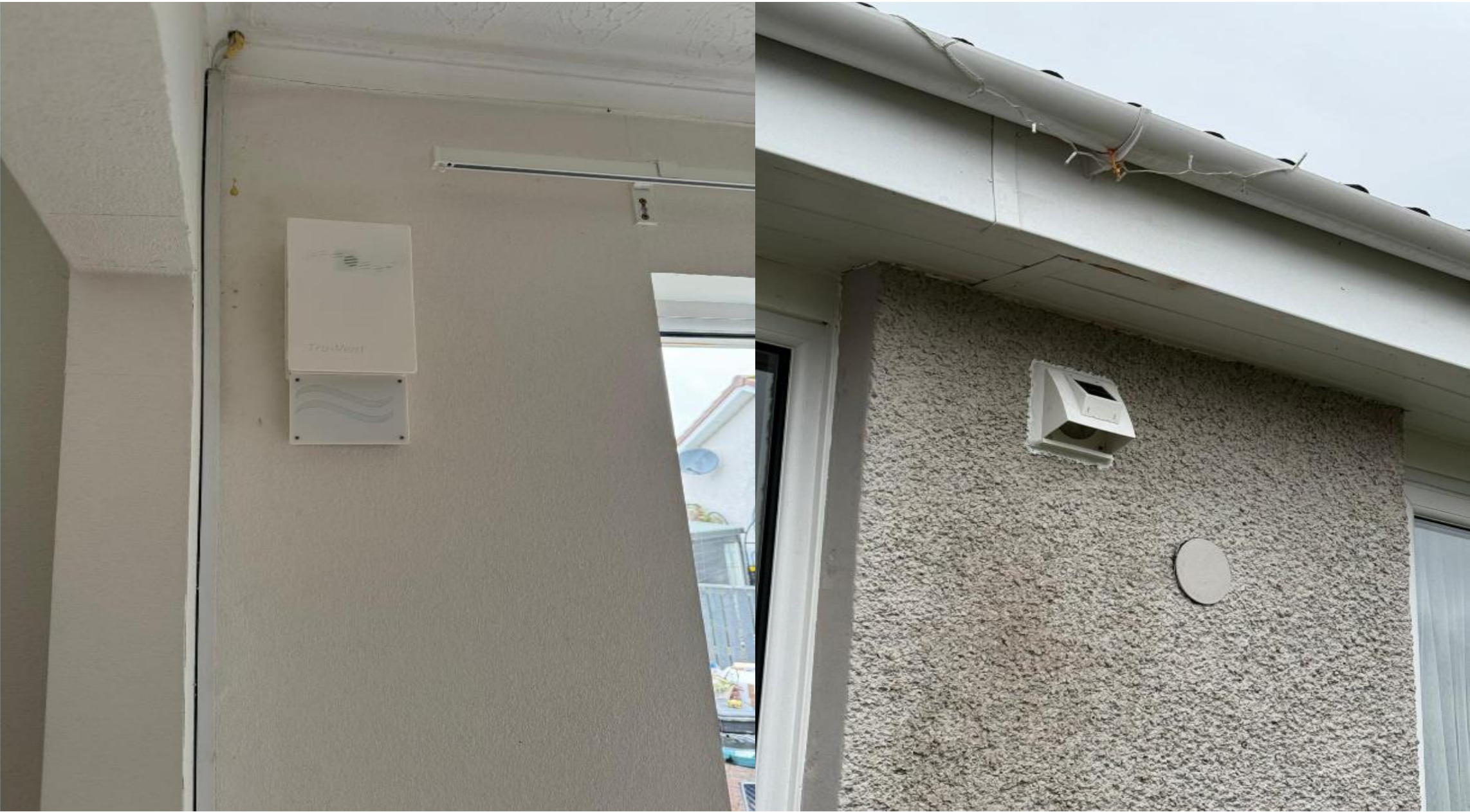
Installation of the passive wall vent from the inside
