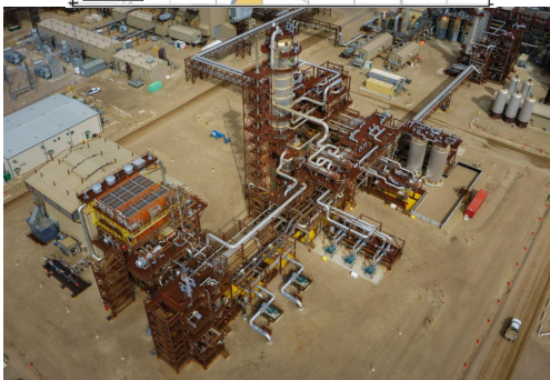
Quest CCS project location and capture facility (Rock et al., 2017)
