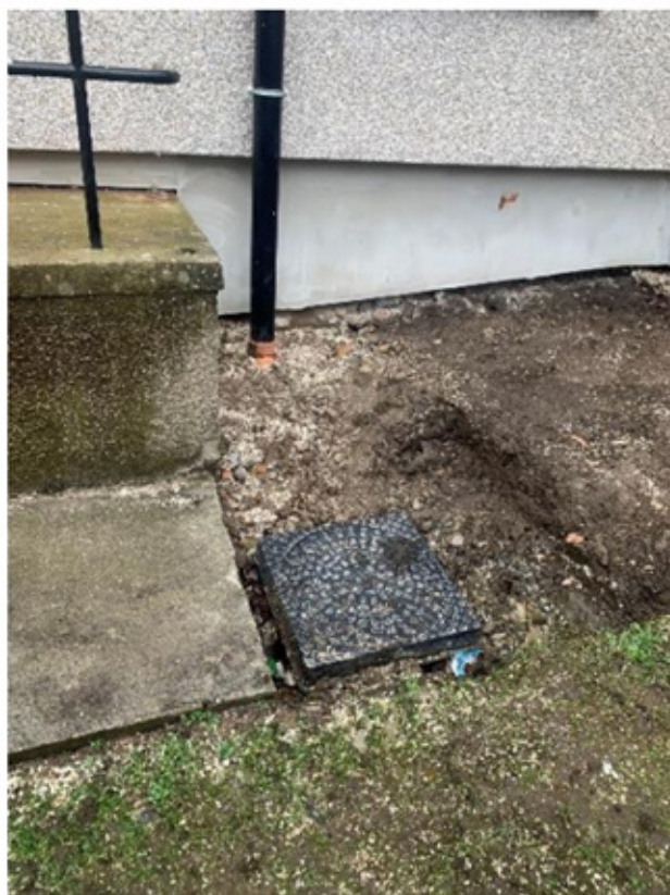
Image: Repositioning of Drainage, Skye Elizabeth Chatburn
