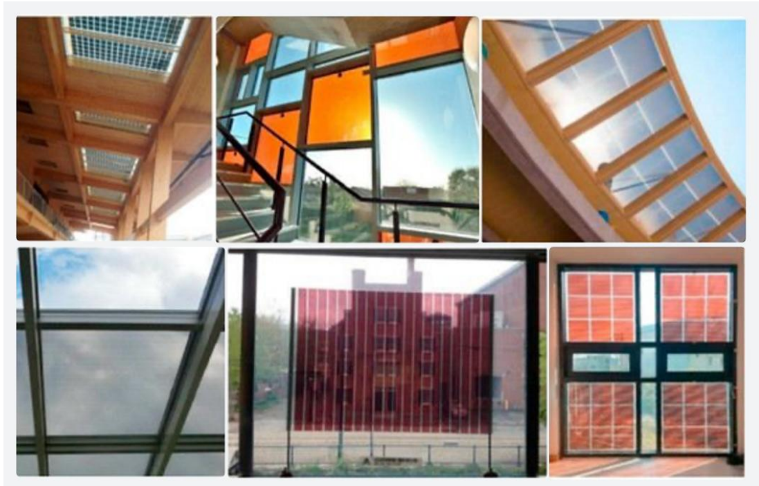
Figure 17. BIPV application with different cell materials (Reddy et al., 2020)
