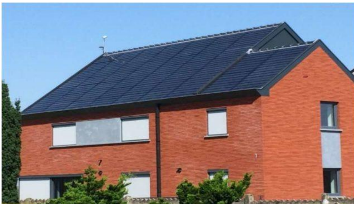
Figure 15. Example of BIPV roofing (Bungane, 2017)
