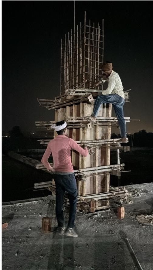
*Figure 6.6: Laying a column in case study 1 (Photograph: Construction Interviewee 2)*
