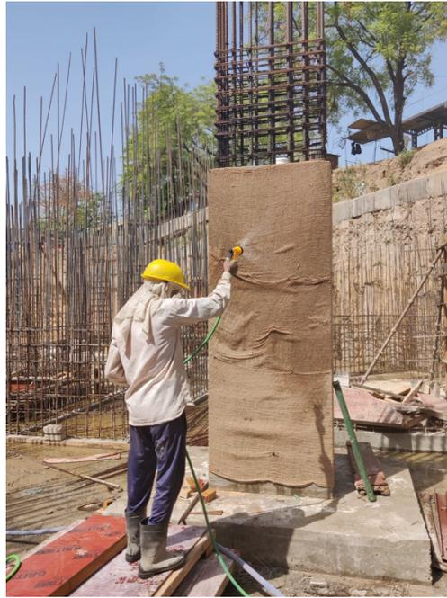
*Figure 7.4: Water management practices followed during column curing during construction of case study 2 (Photograph: Construction Interviewee 2)*
