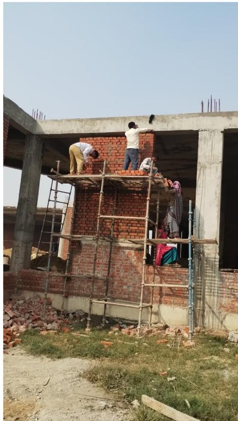
Figure 6.3: RC Frame with clay brick construction (Photograph: Construction Interviewee 2)
