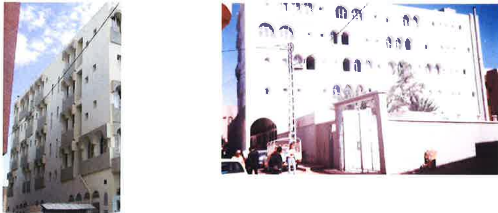
Figure 2. Views of the north-east (left) and the south-east (right) facades of the CNAS building.
