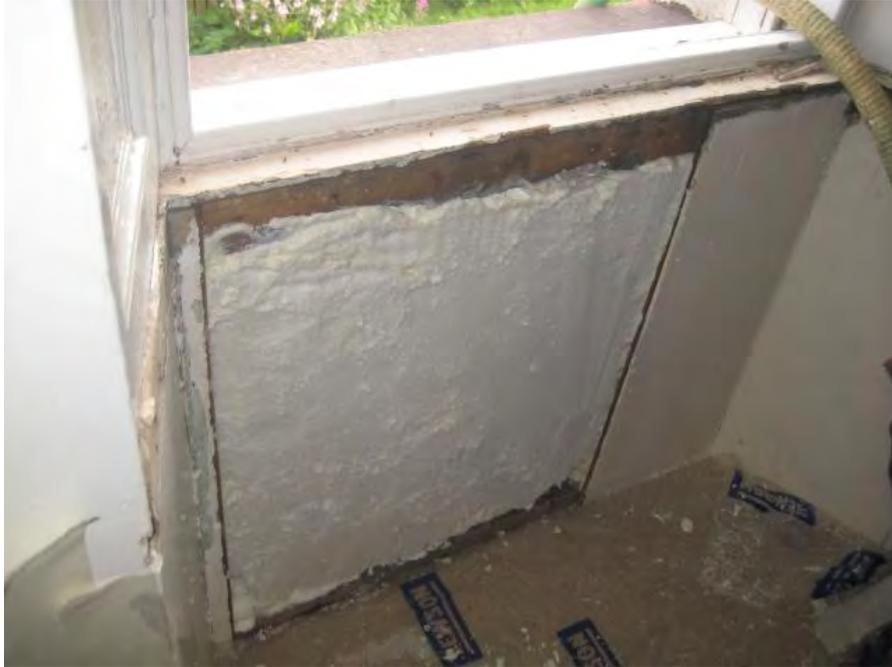
**Insulating the wall under the window**
