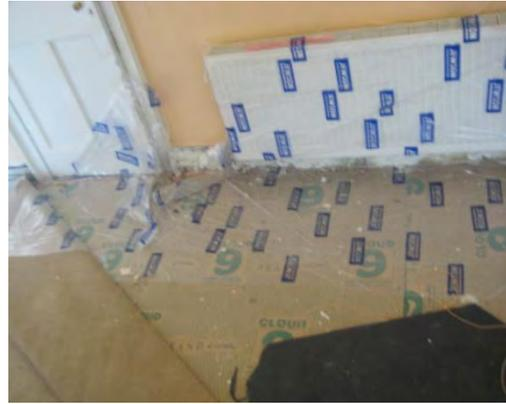
**Covering of the floors, features for projection against the foam that might be damaged by accident**
