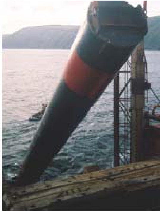
Figure 1-18: 2003, SeaFlow's monopile. (Courtesy of Marine Current Turbines Ltd)
