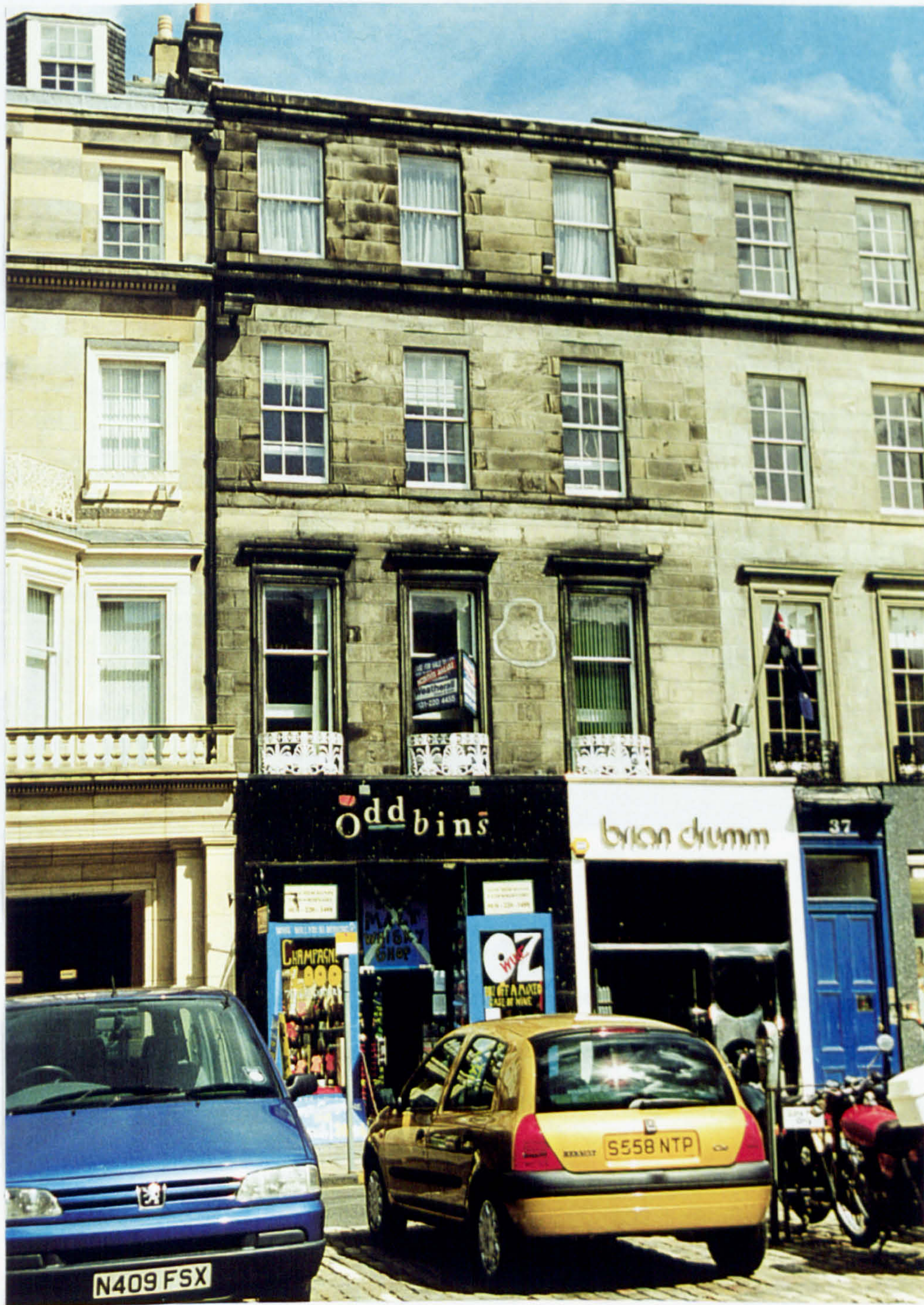
Figure 7.2 - Building selected for example 1
