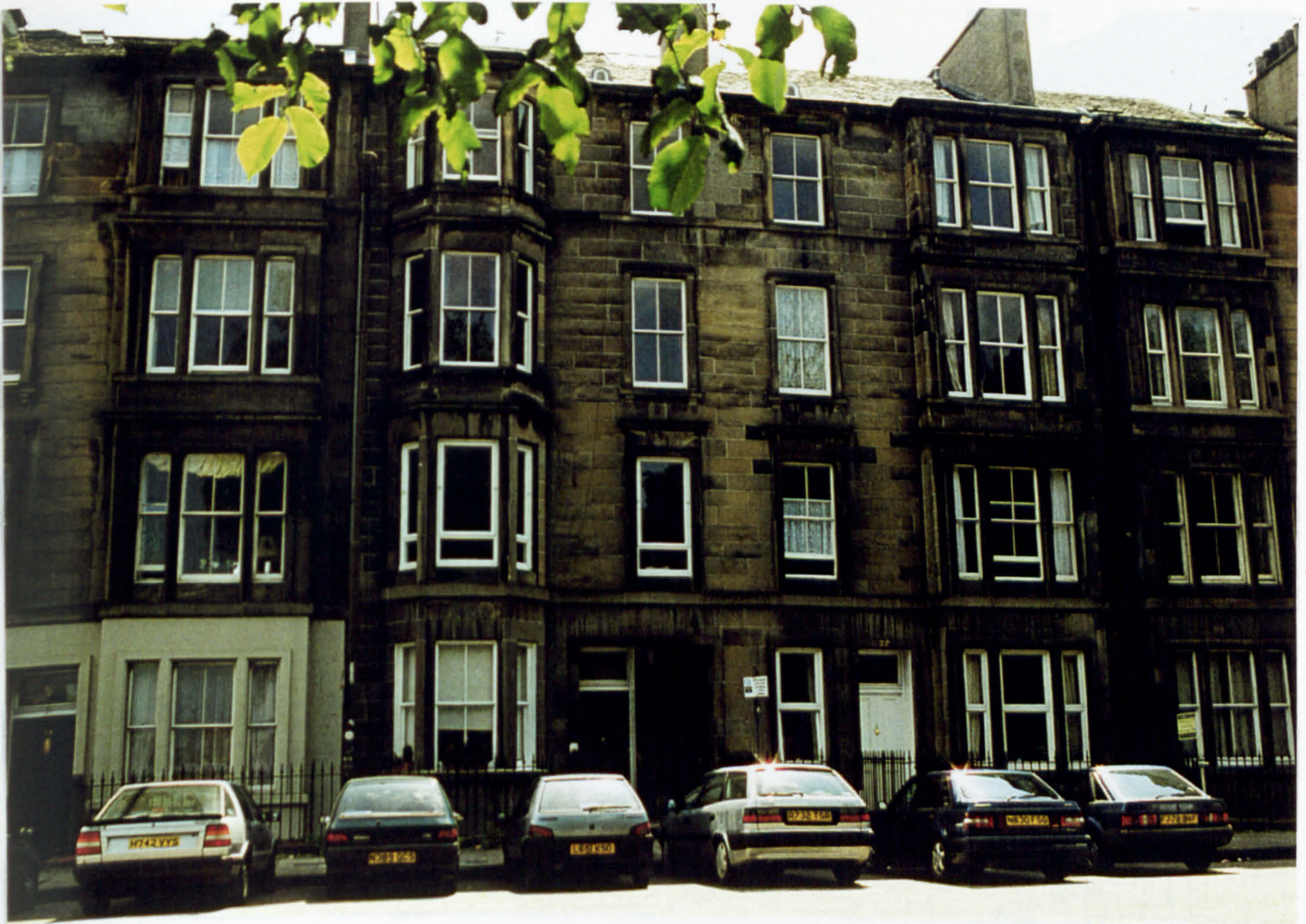
Figure 8.3 - Building selected for example 1
