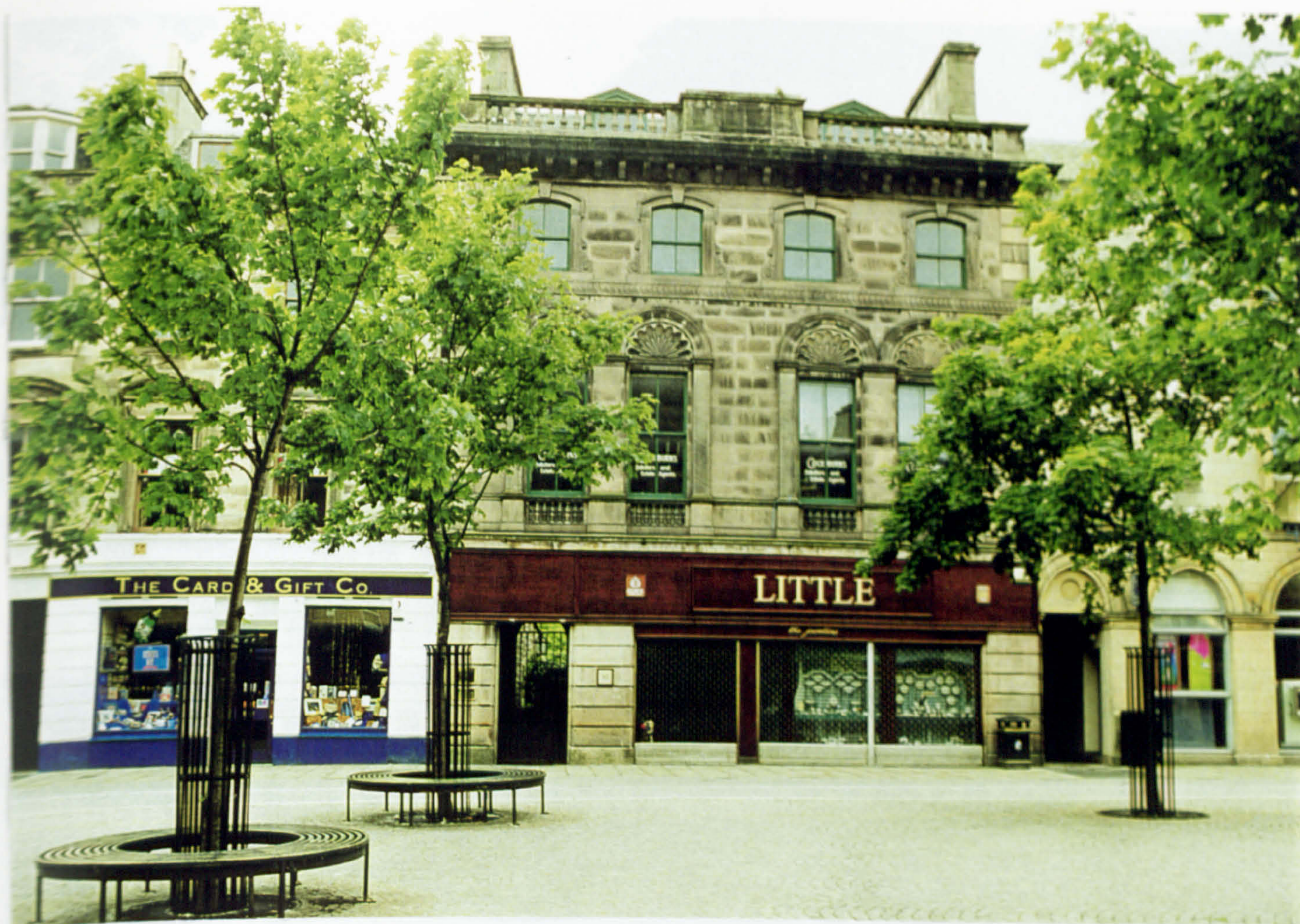
Figure 7.5 - Building selected for example 2
