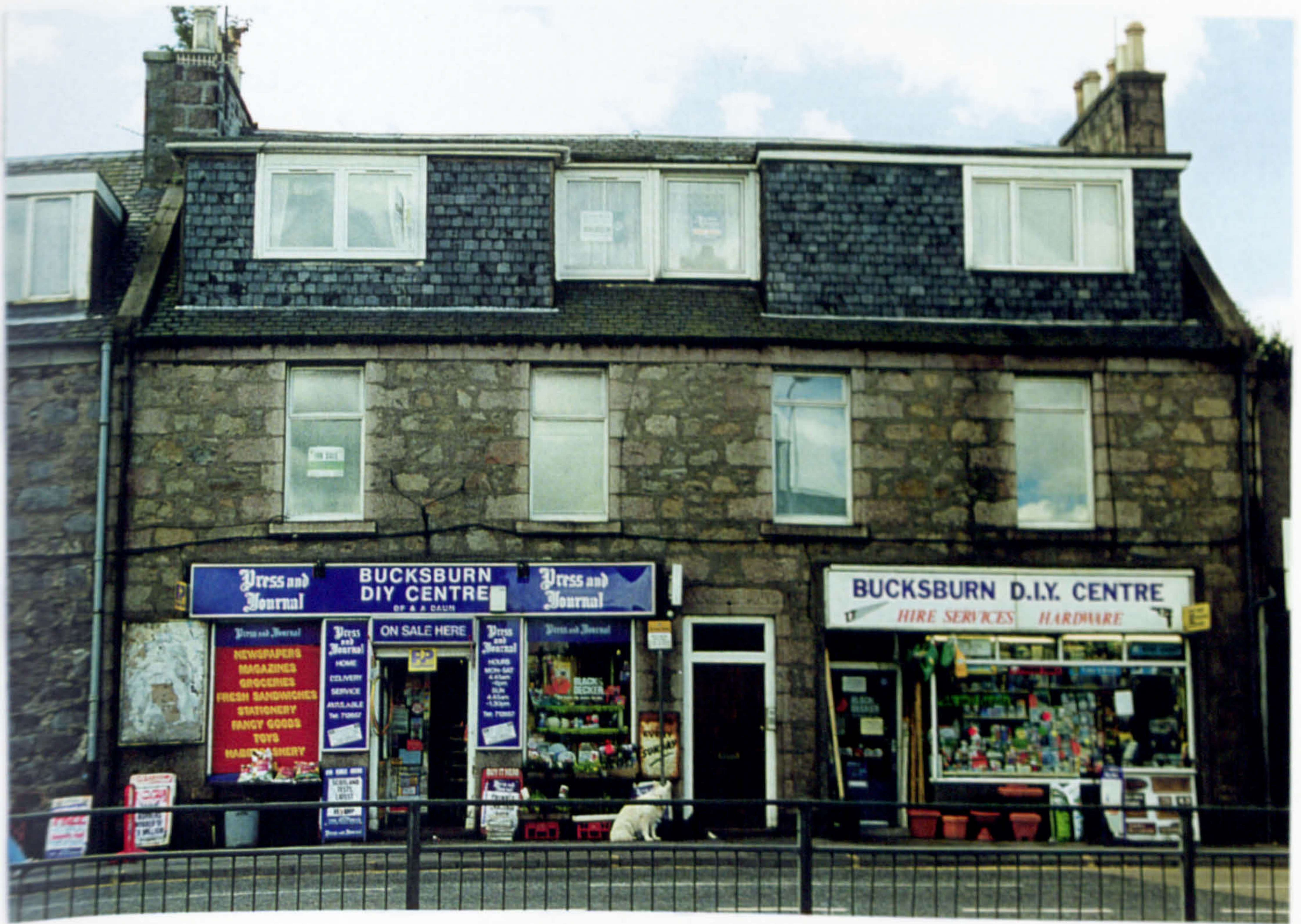
Figure 8.5 - Building selected for example 2
