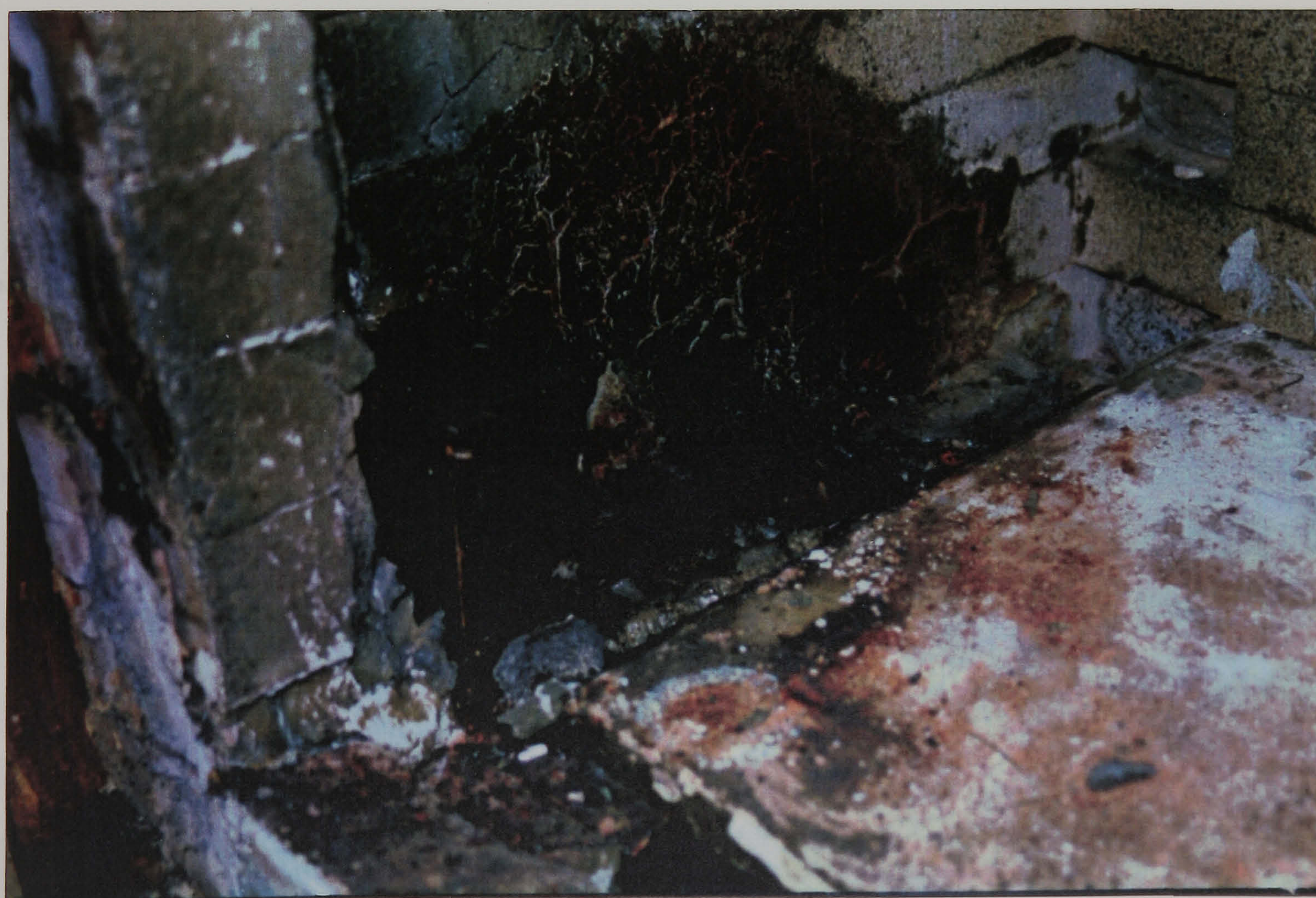
Figure 1.5 Conventional fire bricks showing damage due to alkaline attack.
