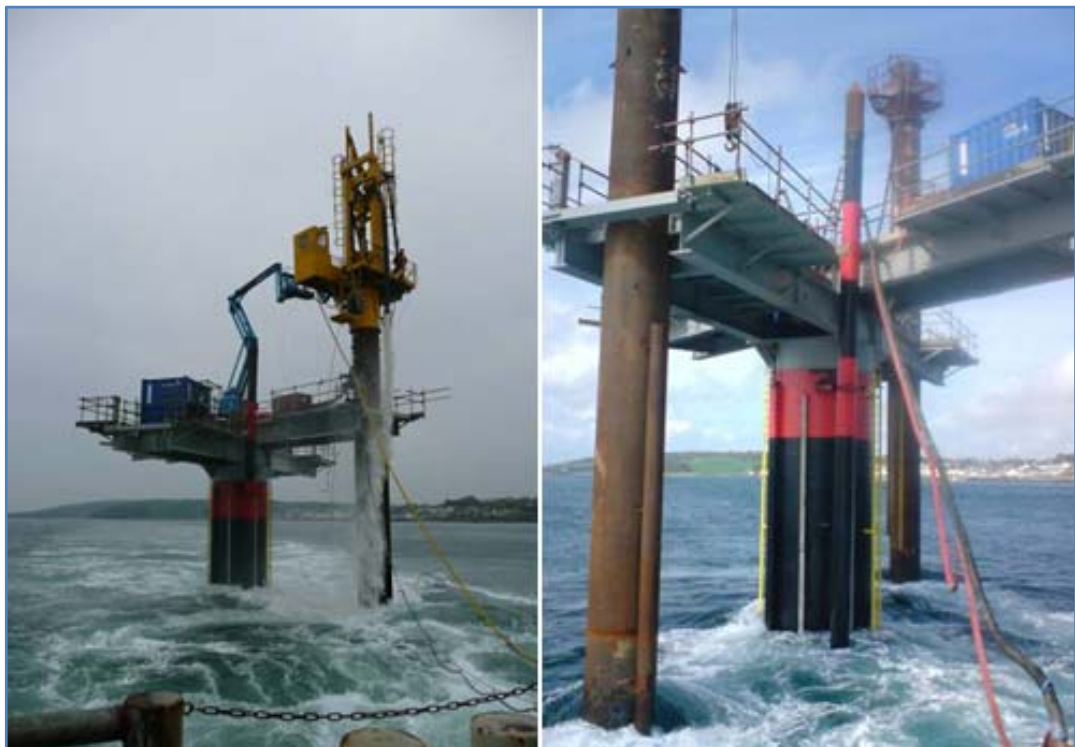
Figure 2.38: MCT Installation Operation (36)
