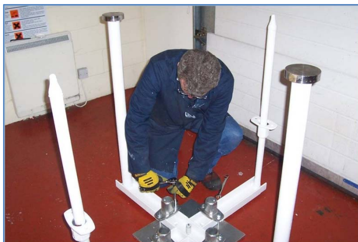
Figure 4.6: Construction of the base support structure, being attached to the base. Magnet locking plates shown (copyright author)
