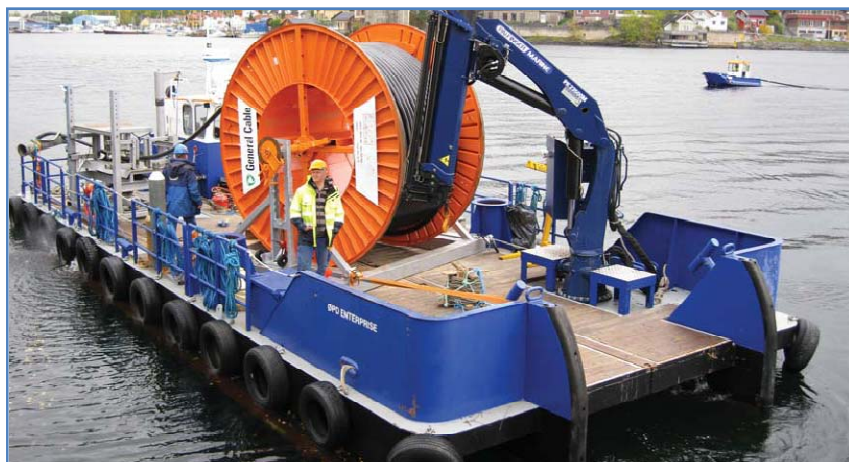
Figure 5.5: Meercat RT16 in harbour cable laying mode (64)
