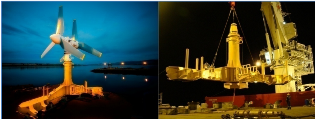
Figure 2.44: AK-1000 turbine on keystone, and support support base structure being loaded aboard installation vessel (45)
