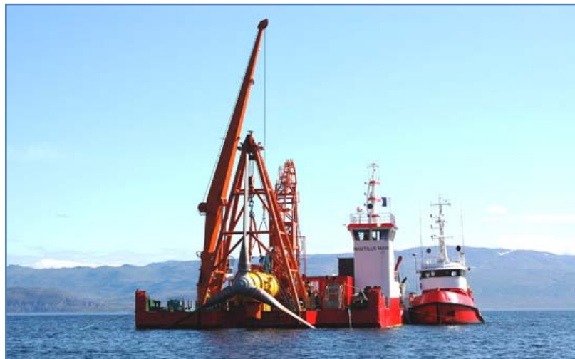
Figure 2.42: A Hammerfest Strom prototype being installed (42)
