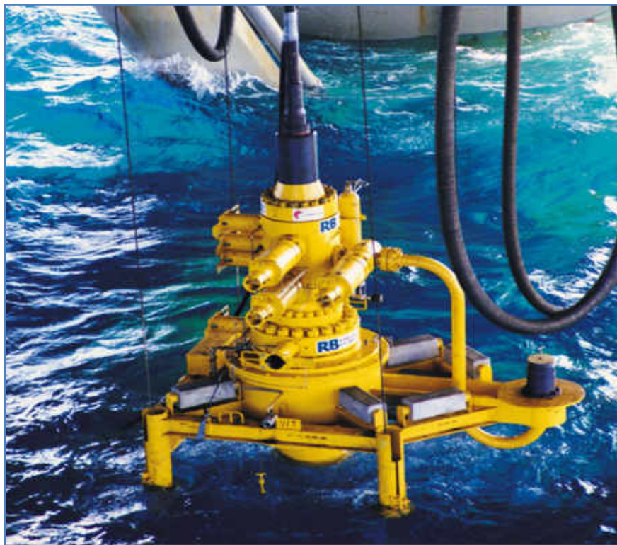
Figure 2.22: A simple subsea tree being deployed from a rig, down the guidewires (20)
