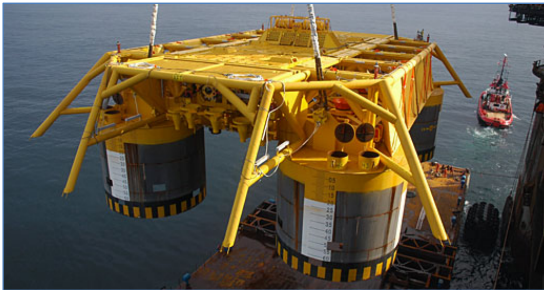
Figure 2.9: Subsea Template attached to four structures (called 'mudcans') to provide stability on seabed (11)
