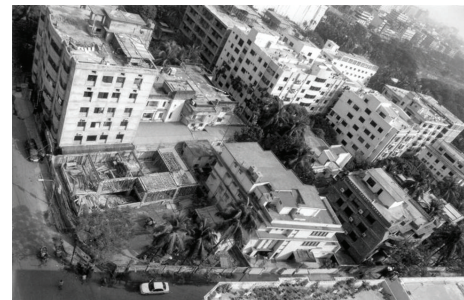
FIGURE 22: Morphology as generated from existing building regulation having FAR 4.2 (Photo credit: Abdullah, 2004).
