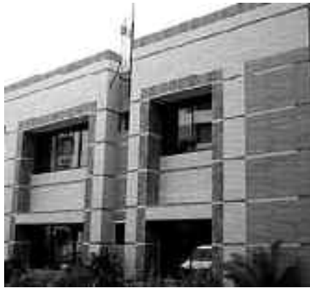
Figure 7. Office converted from residential building (source: STS Holdings LTD.)
