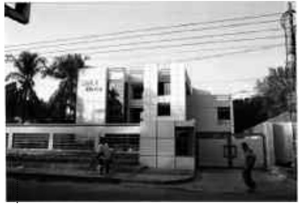
Figure 17. Conversion of the same residential building into corporate office (Mobil House) (source: Mahbuba Haque. 2006)
