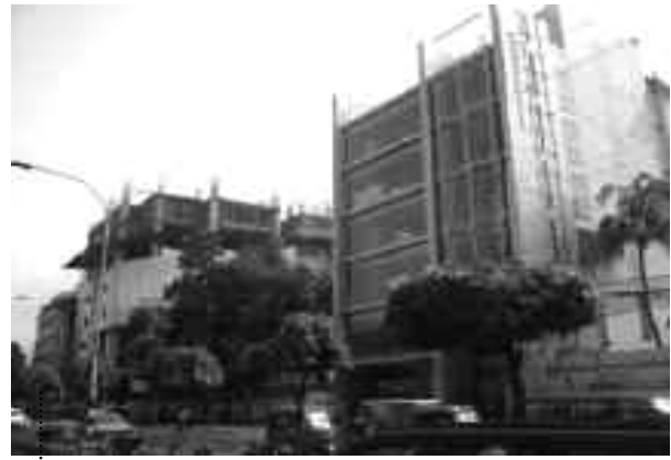
Figure 8. Main road of diplomatic zone is regenerated into commercial zone making a new urban edge condition (source: http://www.skyscrapercity.com , accessed on 28 December 2010)
