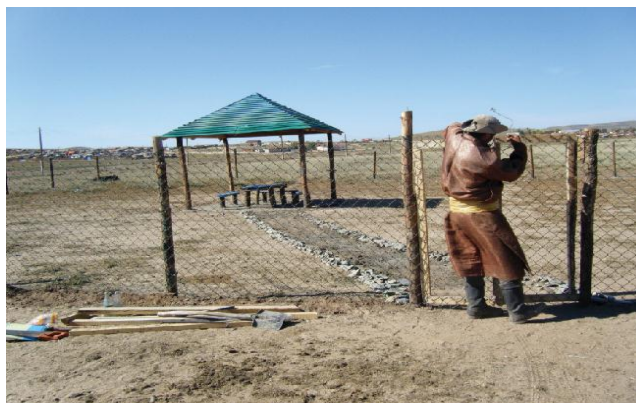
Finishing the making of a gate
