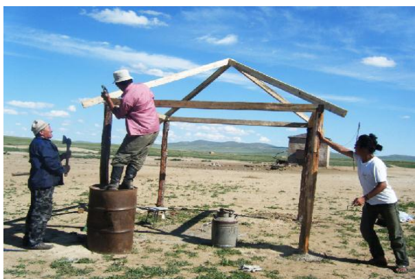
Overall structure of the sunshade
