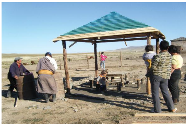
Finishing up the roof
