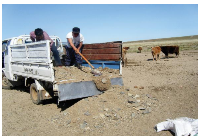
Unloading gravel to level the ground
