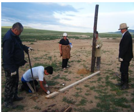
Started to build a sunshade
