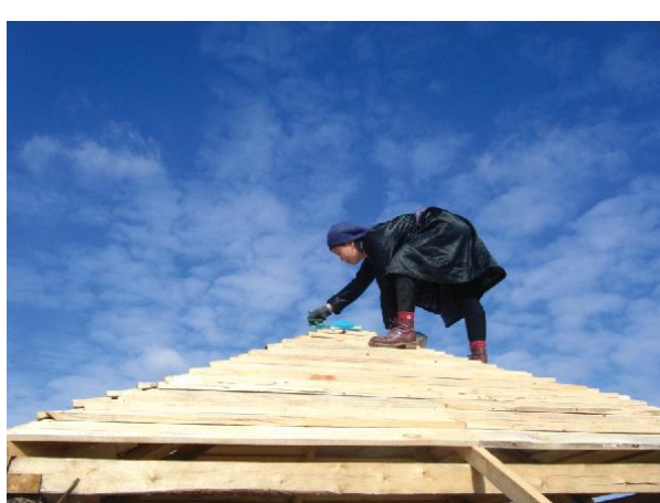
Painting the roof of the sunshade/Munguntsetseg
