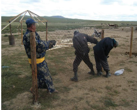
Building a wire net fence
