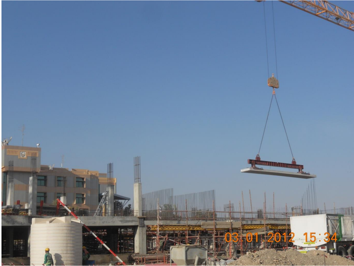
Figure 4.10: UAE university- case study E (Source: Nael General Contracting Establishment)
