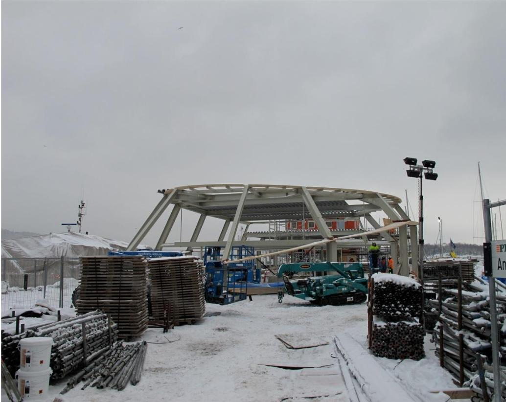
*The structural solution providing post and beam construction. The problem that developed from this solution was that a torque had to be applied to make them flush to the skin.*
