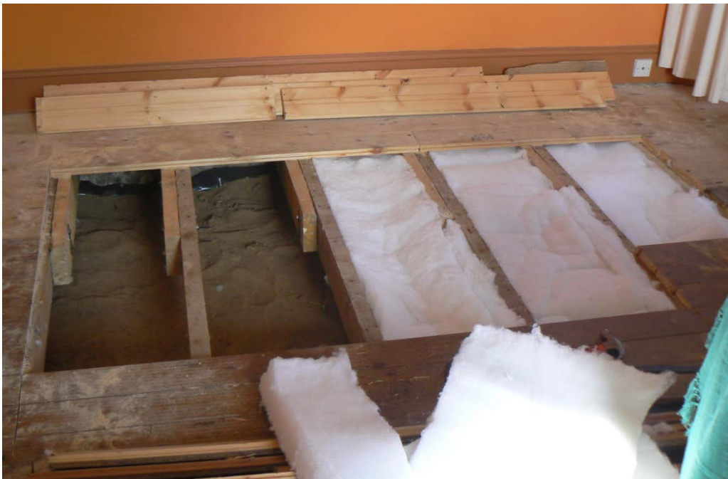
Figure 6. Addition of insulation to suspended timber floor.
