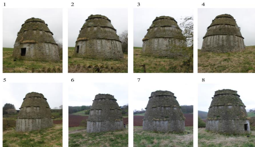
Figure 2. Systematic photographic recording process
