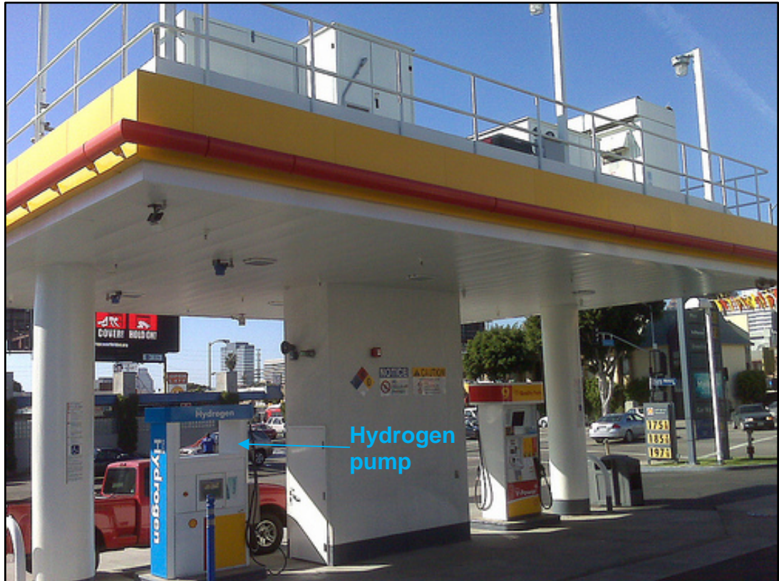
Figure 7: Hydrogen Filling Station (19)
