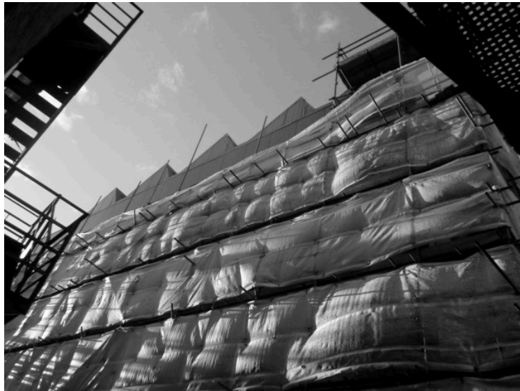
Waygood Gallery. Newcastle upon Tyne, Under construction 2010
