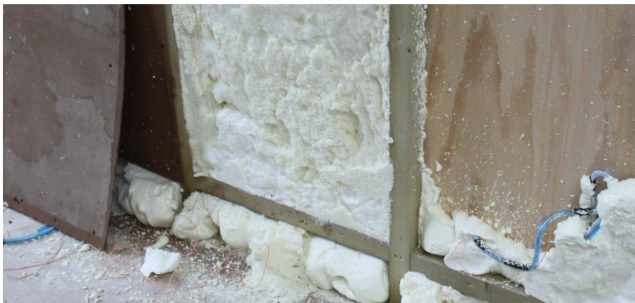
Figure 2-20 Trial application of PUR foam in a narrow cavity (Courtesy of Kishorn Insulation)
