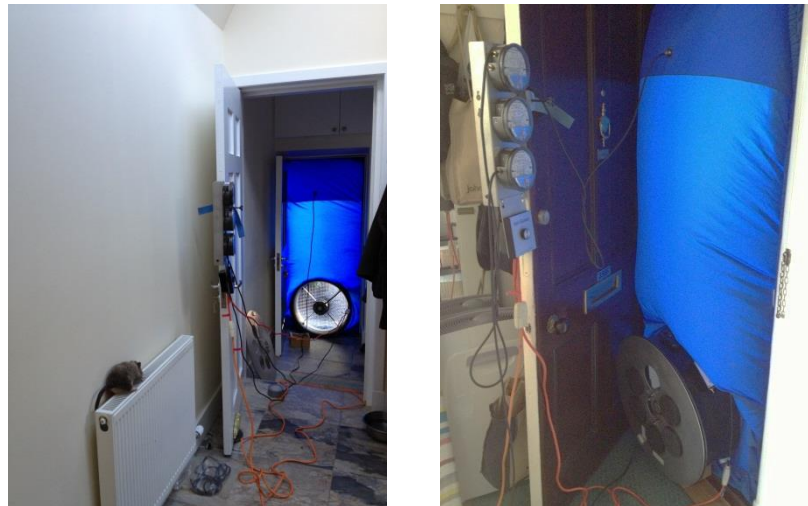
Figure 3-6 Air pressure tests
