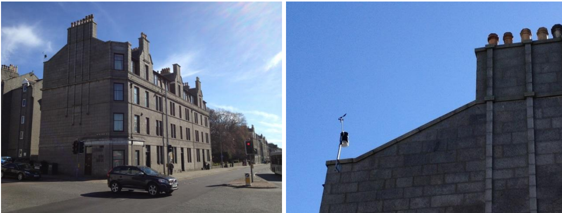
Figure 3-7 The external weather station installed in the city centre of Aberdeen
