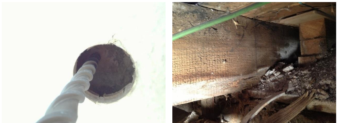
Figure 3-8 Probe installation (left) and floor joist exposed during the survey (right)
