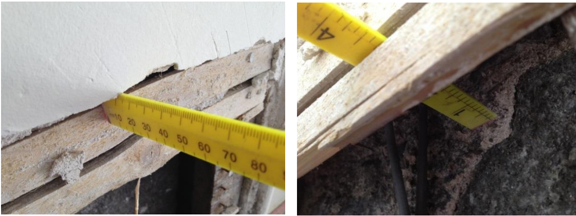
Figure 3-9 Measurements of the internal lining (left) and cavity width (right).
