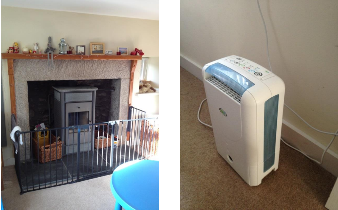
Figure 5-2 Case 13. Wood burning stove in the living room (left) and dehumidifier (right).
