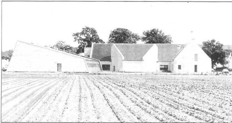
Rear facade of Highland Craftpoint, showing the workshop wing on the left hand side.
