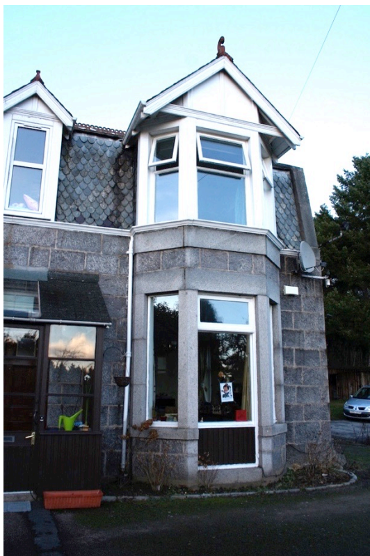
Figure 2: 'Ouch!' Negative impact of drastic change in window types. (Milltimber, Abd.)
