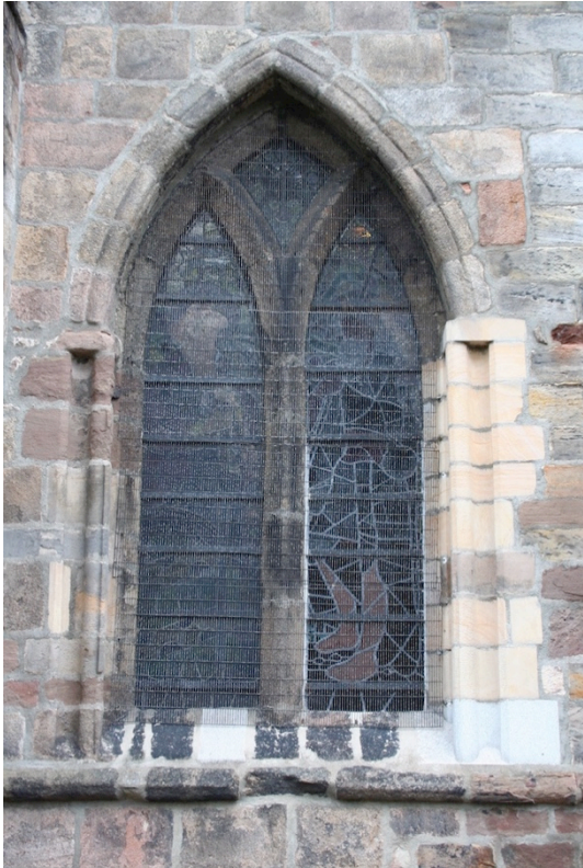
Figure 1: 'Ouch!' Repair creating attention-drawing contrast. (St. Machar's Cathedral, Aberdeen)
