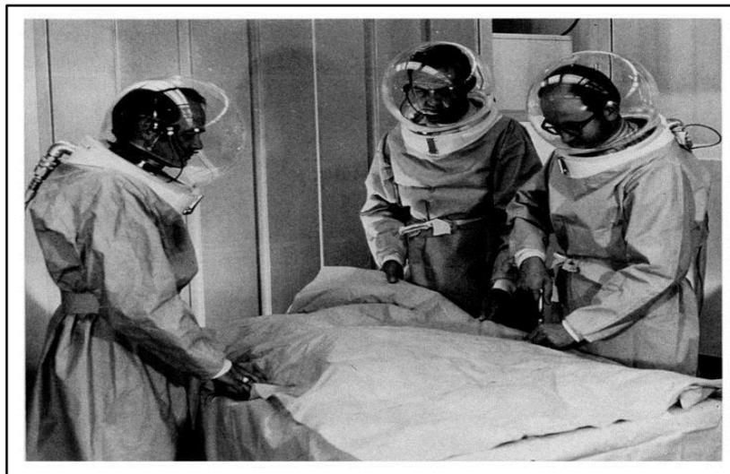
**Figure 1 – 1:** Surgeons working in a clean room at St. Luke's Hospital Denver in 1972. Clean conditions and specialist clothing were used to lower the risk of infections during surgery. Both the room and the clothing were based on space program experience and were developed under NASA contract by the Martin - Marietta Corporation (Taken from: Bilstein 1989) (NASA Imagery – not copyright protected).
