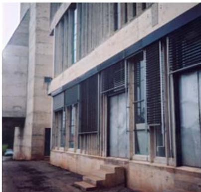
Figure 8. The vertical mullions on the southern façade of the Tourette Convent are ineffective for solar control and users supplant them with venetian blinds [32].
