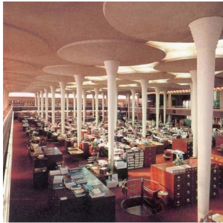
Figure 3. Johnson Wax's office space is provided with zenith daylighting through tubular glass surfaces [12].
