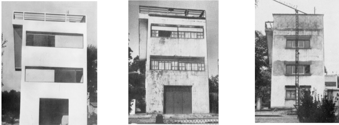
Figure 7. Views of the facades showing their initial state, the addition of curtain blinds for solar control and then the narrowing of the windows [30].
