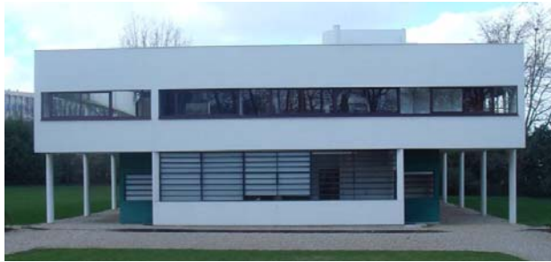
Figure 10. The venetian stores used to protect the windows of the south-oriented manager's office in the Villa Savoye [33].
