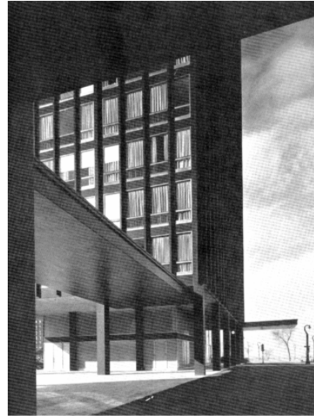
Figure 2. The transparency of Mies van der Rohe's Lakeshore Drive apartments' facades is greatly reduced because of the occupants' use of the external solar protections [6].
