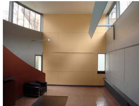
Figure 11. The internal 'brise-soleil' used inside the exposition-reception room in the Villa Laroche [33].
