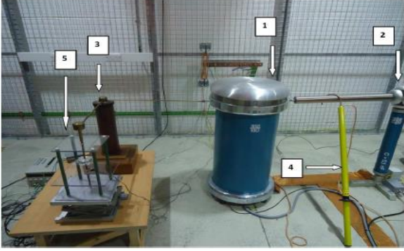
Fig. 1: Photo of the HV system; (1) HV transformer (2), AC capacitor, (3) PD measurement capacitor, (4) Earth rod, (5) Test cell.
