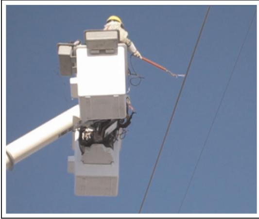
**Figure 1.** A lineman conducting maintenance near energized lines using a hot-stick.
