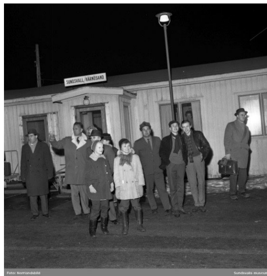
Figure 8: Terminal building at Sundsvall-Härnosänd Airport, used until 1961, courtesy of Sundsvalls Museum
