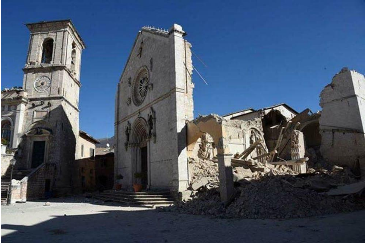
Figure 2. Basilica of St. Benedict collapsed after the earthquake, Norcia, 2016.
