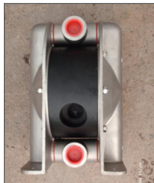
Figure 4-26 shows a 1 inch air operated diaphragm pump installed on SWTS01.
