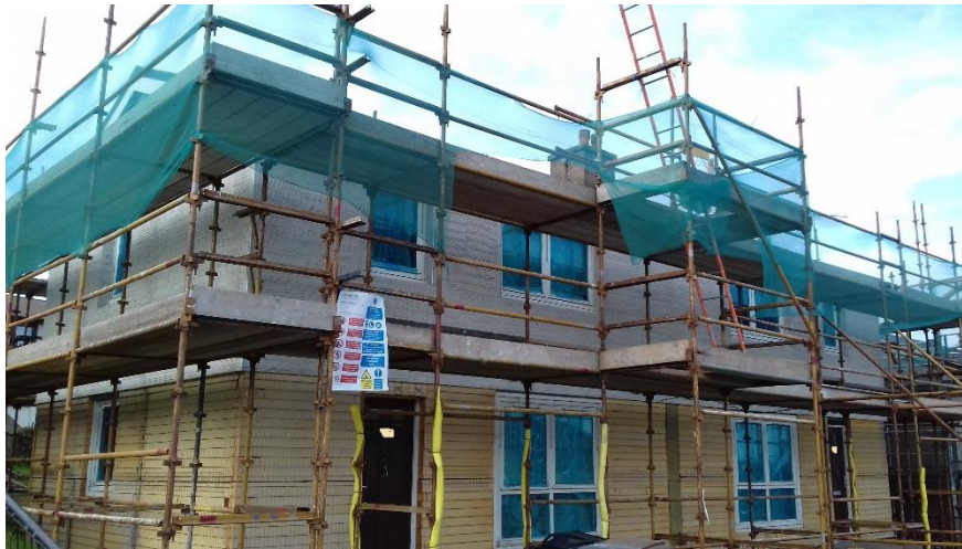
Figure 8: BISF house during external wall insulation (EWI), source: author
