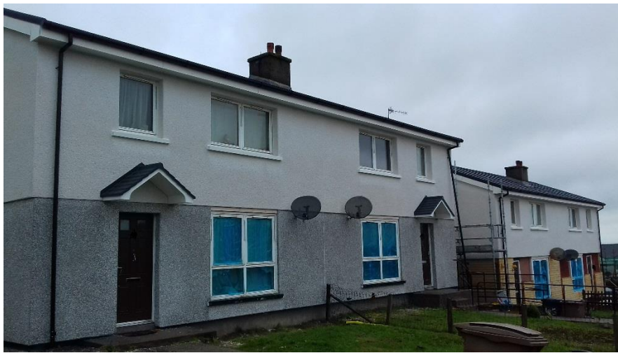
Figure 9: BISF house after retrofitting EWI, source: author
