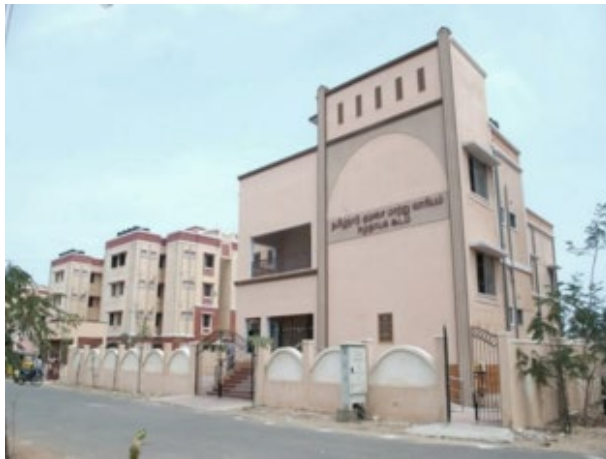
Figure 5 - Community Hall by TNSCB in Thiruvottiyur, India (Tamil Nadu Slum Clearance Board, 2017)
