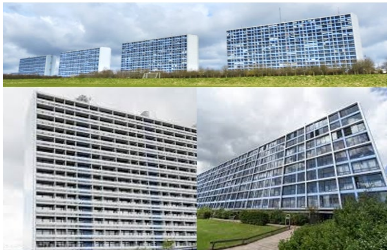
Figure 2: At the top the Hoje Gladsaxe tenement buildings as they appear today. Below are two images showing how they looked at both main facades before and how they now look much newer after the refurbishment of the park facade. Google Earth, 2019
