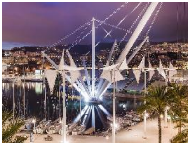
Fig.17 Bigo elevator. Genoa harbour
