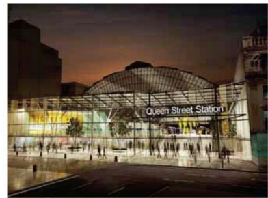
Queen Street Station, Glasgow, UK (BDP)
