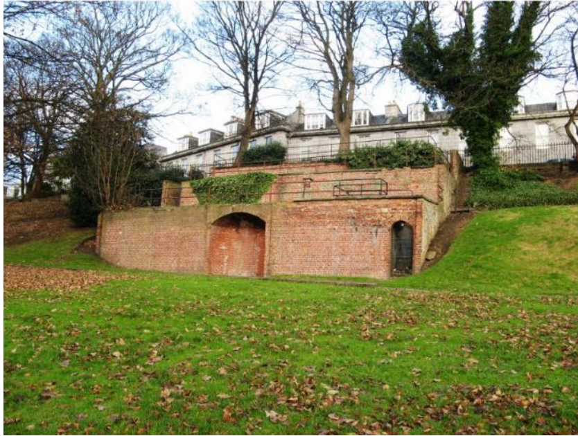
Fig.111: Bon Accord area and garden, view of the terraces
