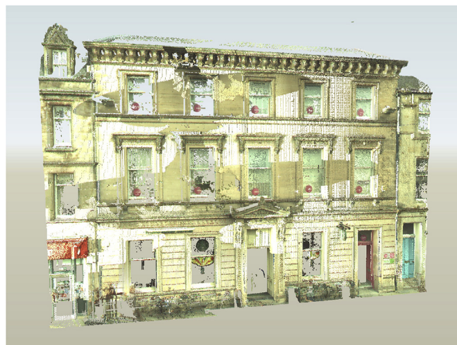
Fig. 2. Example from laser scan of protected building in Elgin, Scotland (scan undertaken by Dr Marianthi Leon).
